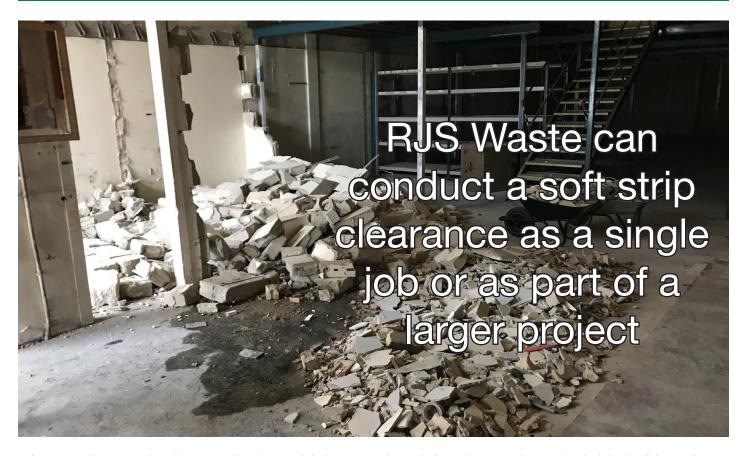
Soft strip works are conducted prior to demolition, refurbishment or remodelling of a building. The intention is normally to leave nothing but the steel frame/shell and involves removal of all non-structural elements of the interior and exterior, including:
